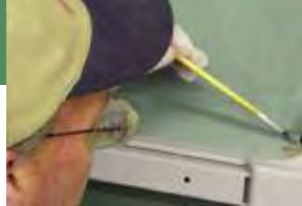
Painting a tight area on a steel door with a Marking Brush.
