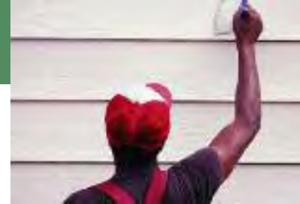
Applying paint to clap board siding.
