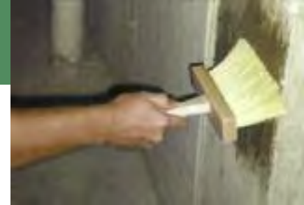
Applying waterproofing material with a masonry brush.
