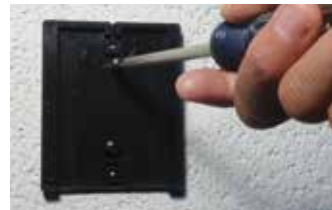
Attach Plate to Wall
